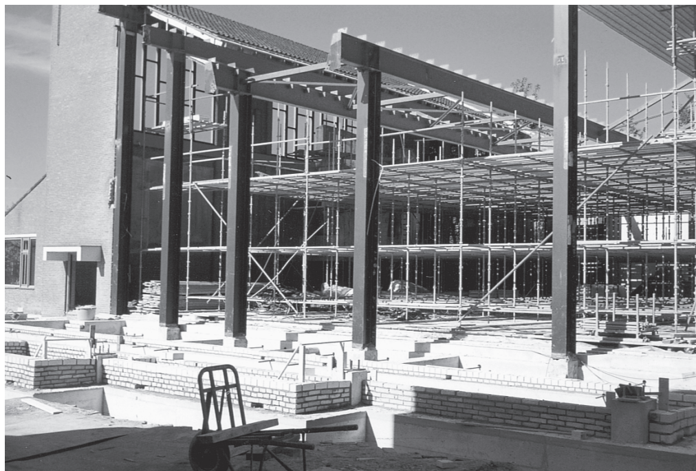
De verbouwing is in volle gang.
